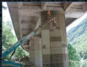
**Hydro-demolition of parts of laminated, fessured or damaged, revived with hydro sandblast of all remaining surfaces.**
